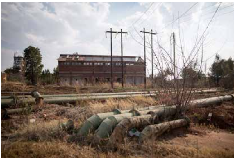
Abandoned Mine building near Mine Shaft 4.
